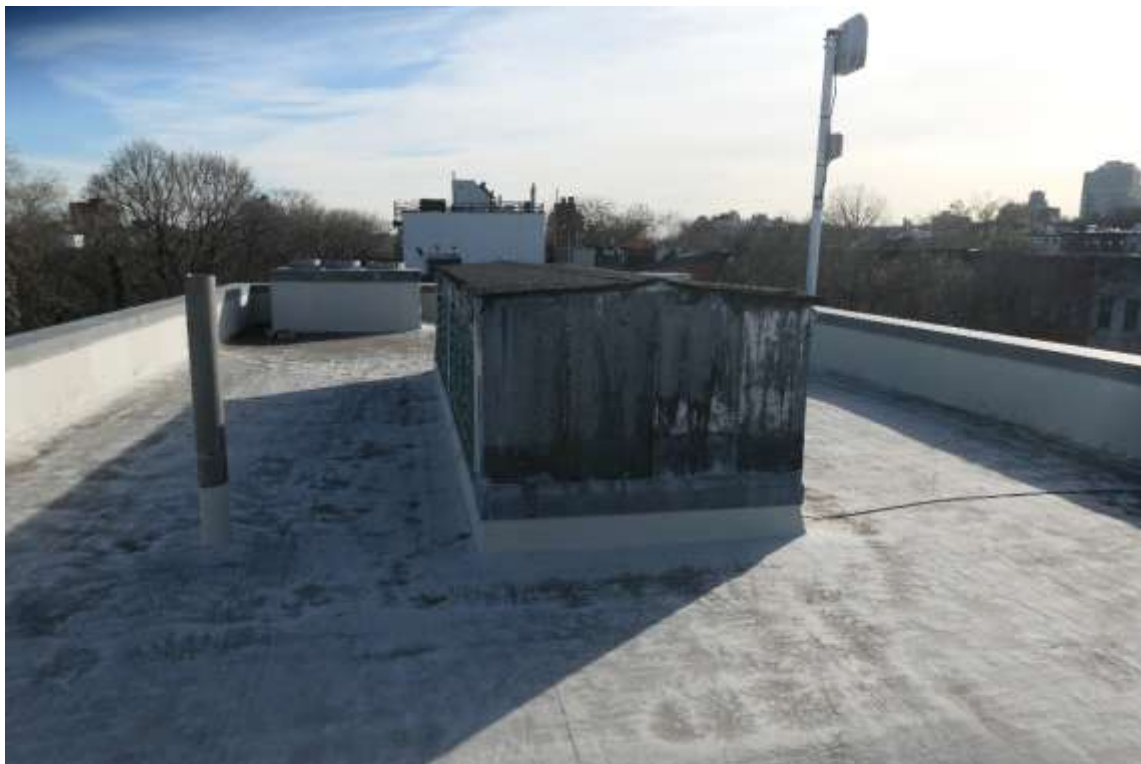
Photo R14 – View of bulkhead roof facing East.
