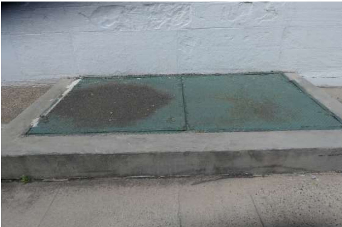
Photo S04 –Vault/Hoist Doors are in fair condition.
