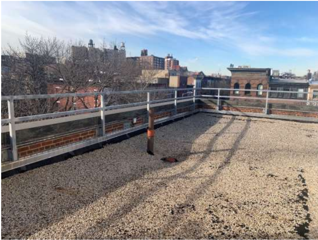
Photo R03 – View of Roof, facing Southwest.
