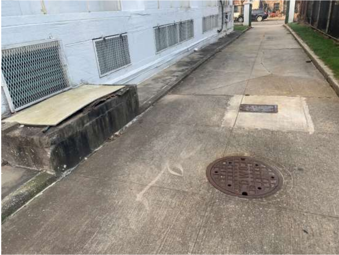
Photo S09 – Areaway located at the north of the building, next to driveway.
