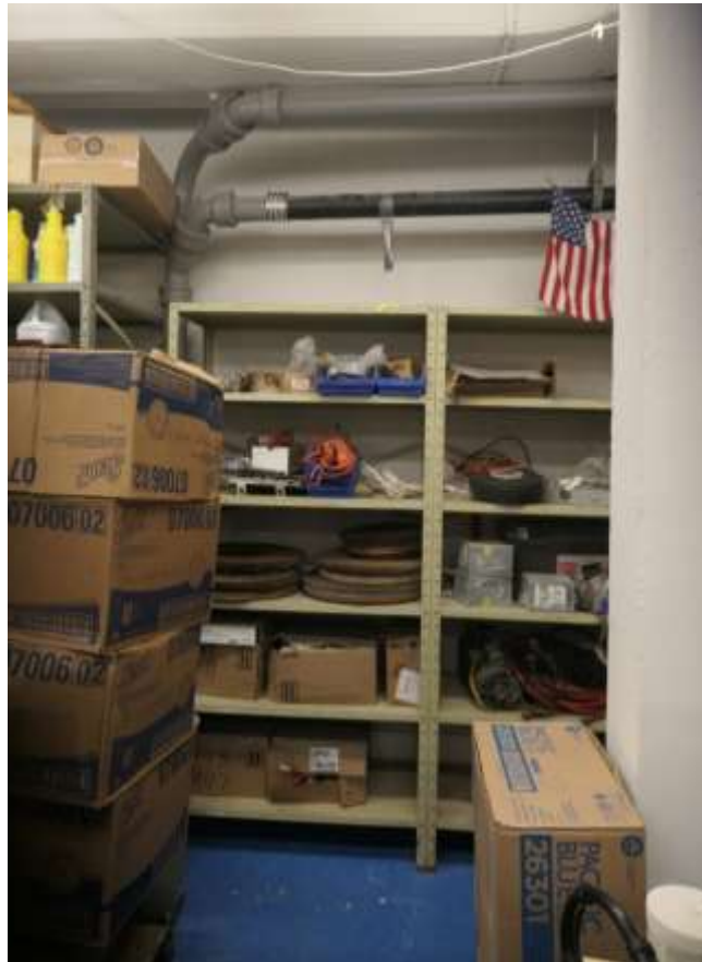
Photo A15 – View of Storage Room B4, view along the wall where the source of infiltration is located.
