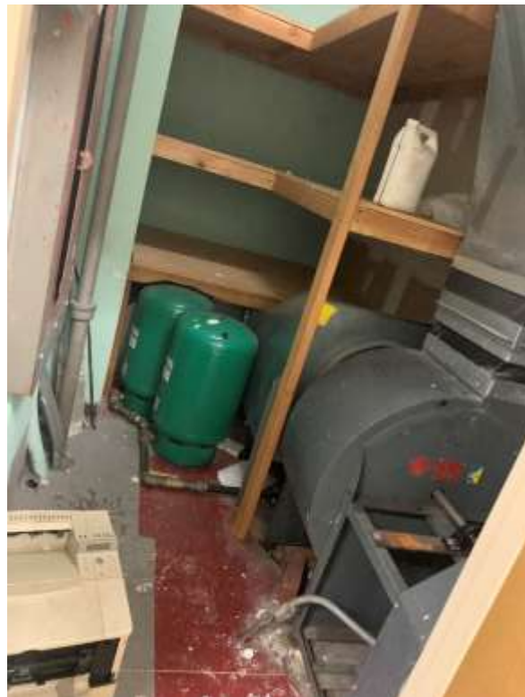
Photo A35 – View of Storage Room at Bulkhead.
