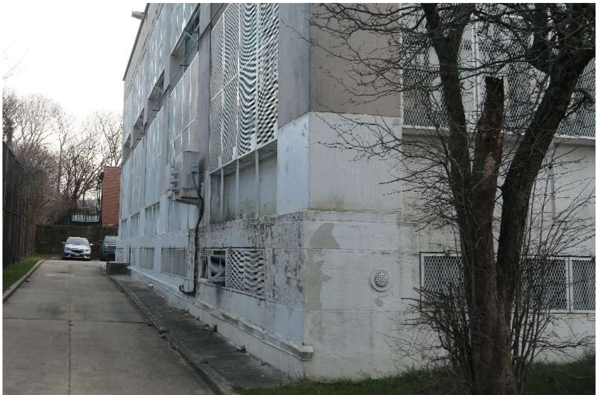
Photo M40– Northwest corner of the building.
