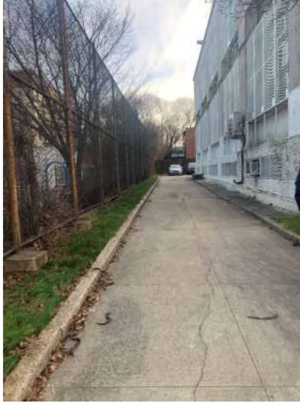
Photo M41 – View along back entrance and parking lot – North Façade.
