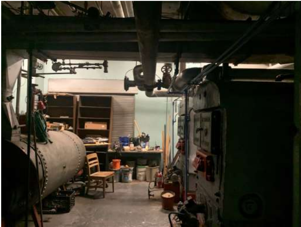
Photo A21 – View of Water Room B7B.
