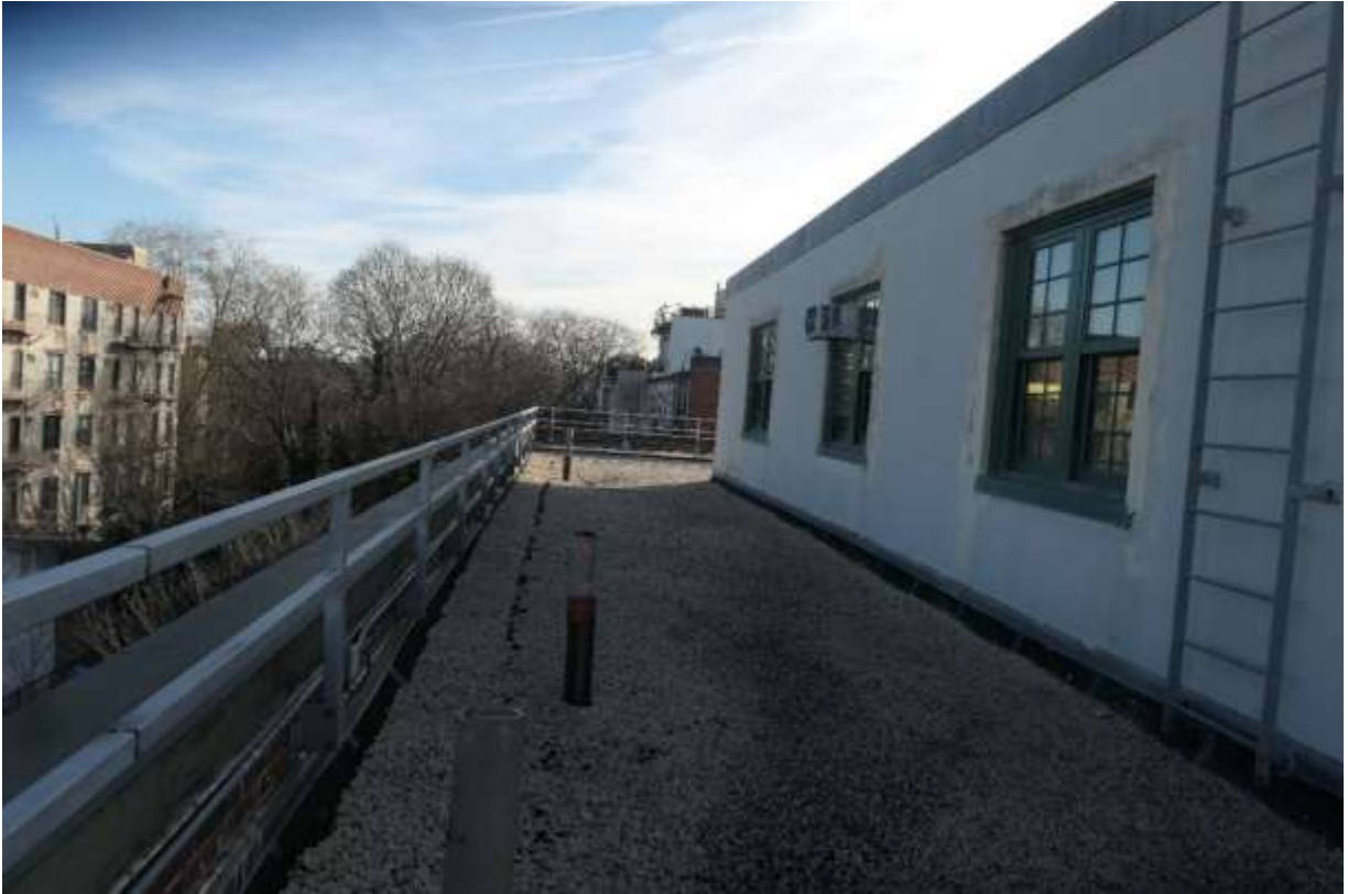
Photo R07 – View of Roof and North Bulkhead façade, facing East.
