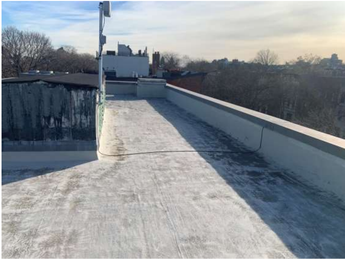
Photo R15 – View of bulkhead roof facing East.
