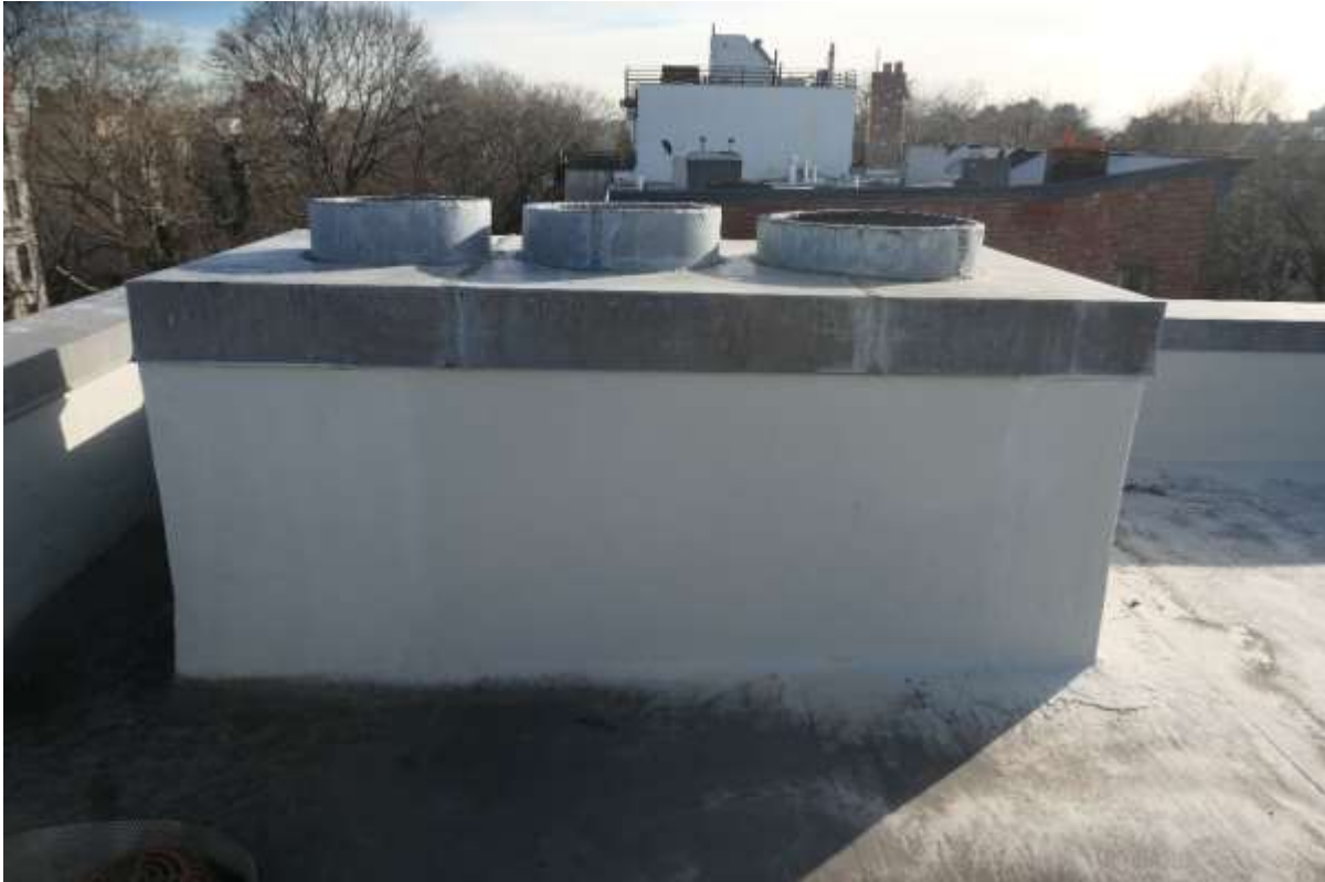
Photo R19 – Chimney at bulkhead roof is in good condition.
