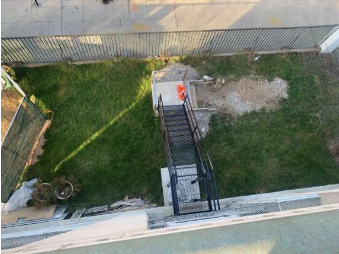
Photo S03 – View of temporary exterior stair at West Façade, taken from Roof.
