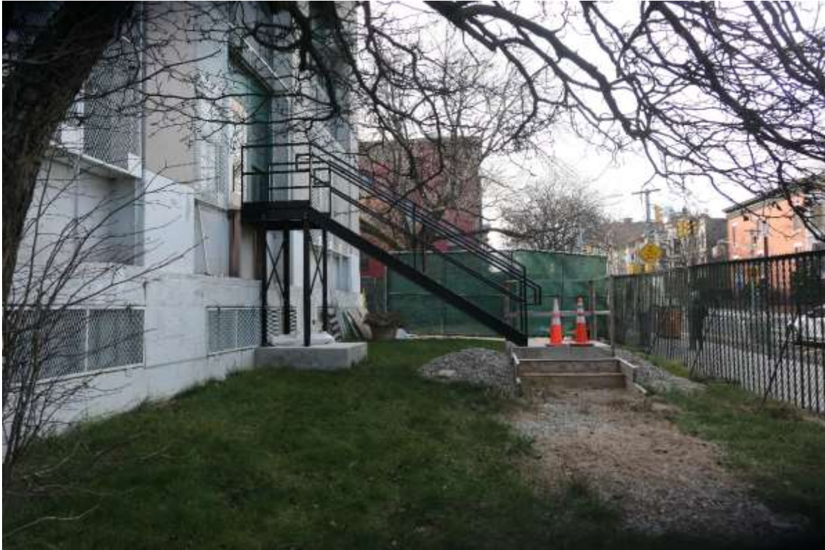
Photo M45 – Temporary stair access at West Façade.
