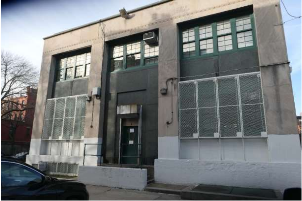
Photo M21 – View from parking lot – East Façade.
