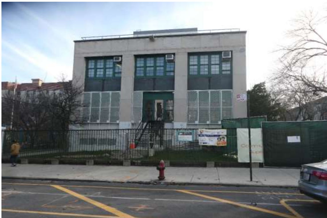
Photo M42 – View along Underhill Avenue – West Façade.
