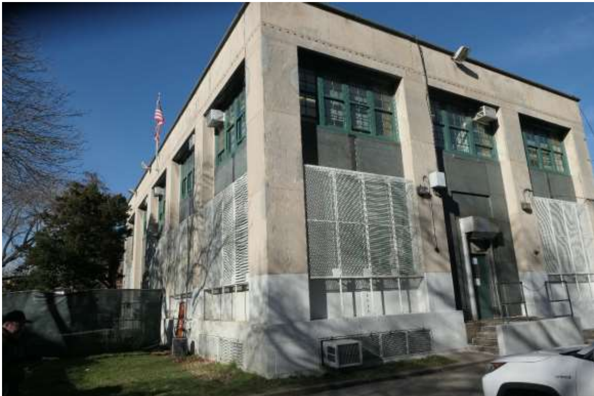
Photo M20 – South and East facades.
