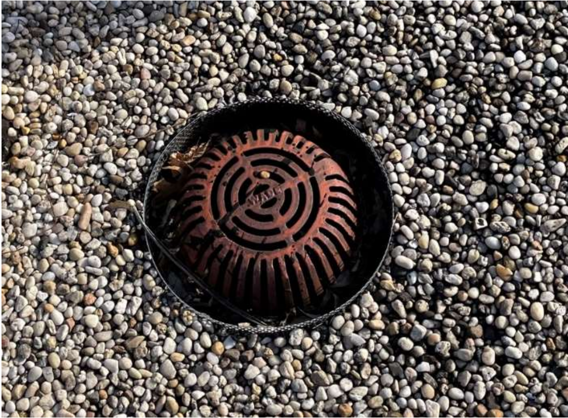
Photo R01 – All roof drains are in good condition.
