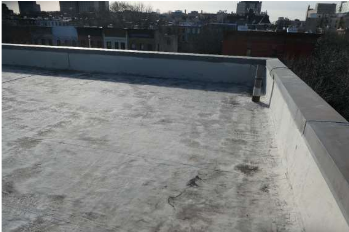
Photo R12 – Bulkhead parapets are in good condition.
