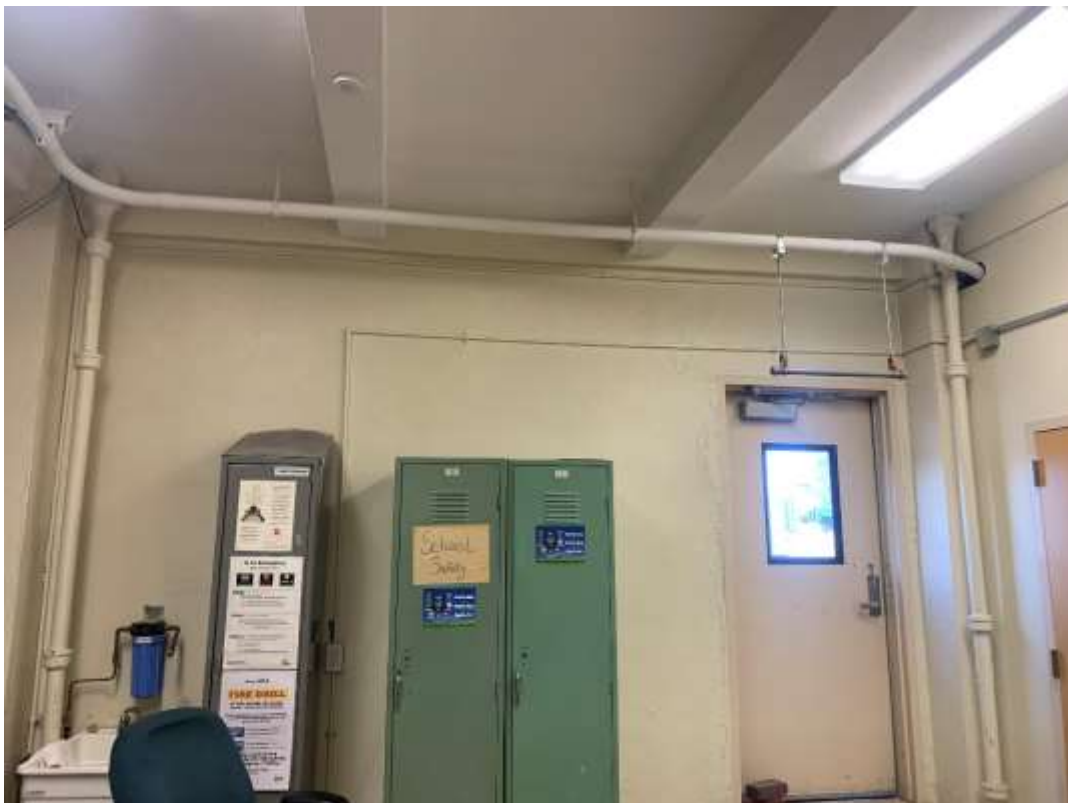
Photo A33 – Bulkhead door – West Façade.
