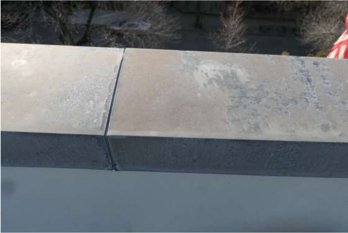
Photo P09 – Parapets at bulkhead roof are in good condition.
