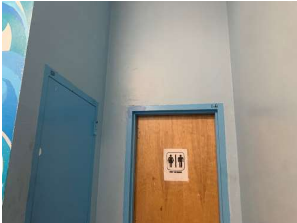
Photo A12– Door to Women’s Restrooms B6.
