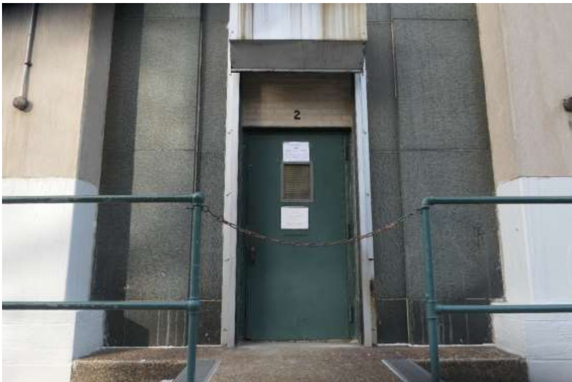
Photo M26 – Secondary entrance at East Façade.
