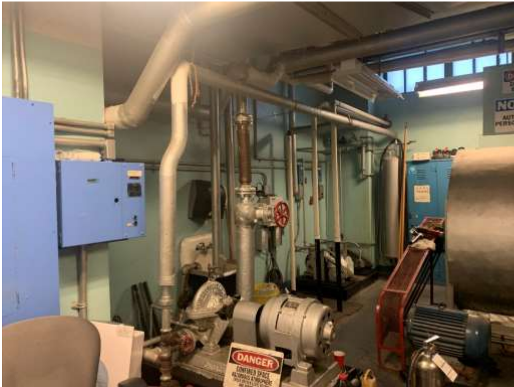
Photo A19 – View of Boiler Room B7A.
