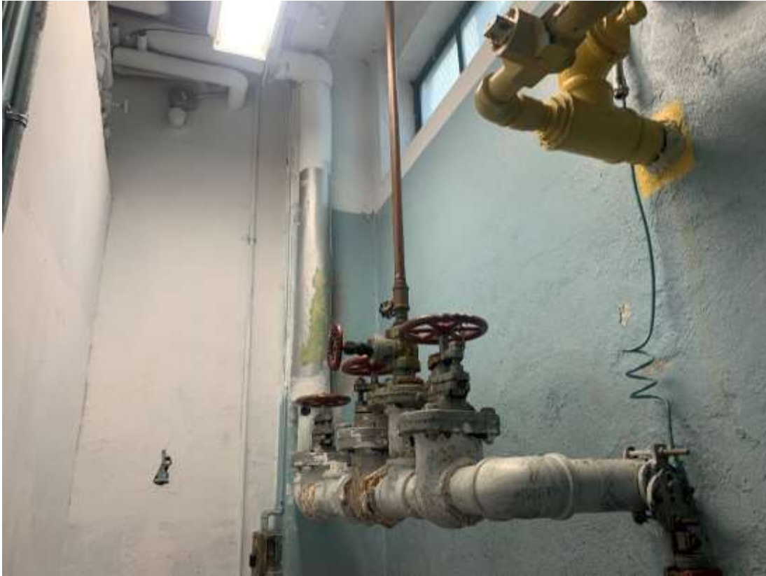
Photo A30 – View of damage at wall in Storage Room B3C.
