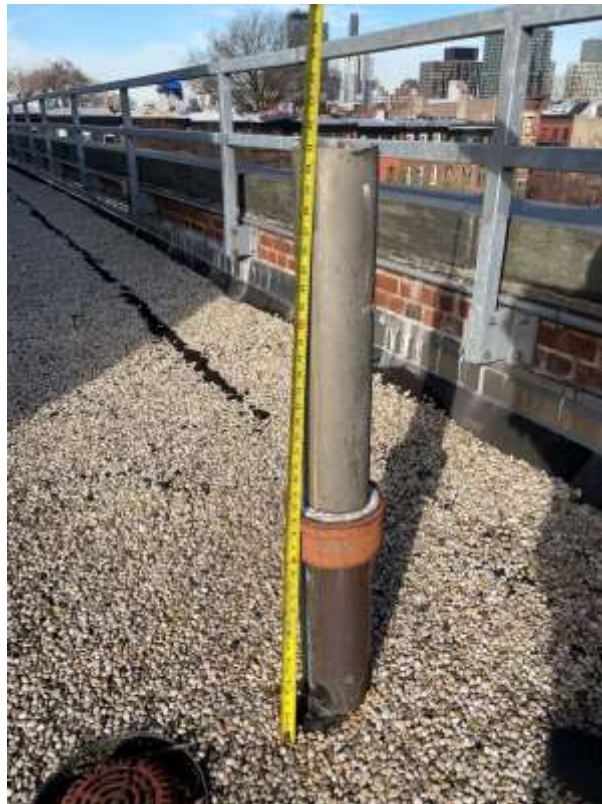
Photo R02 – All vents are in good condition.
