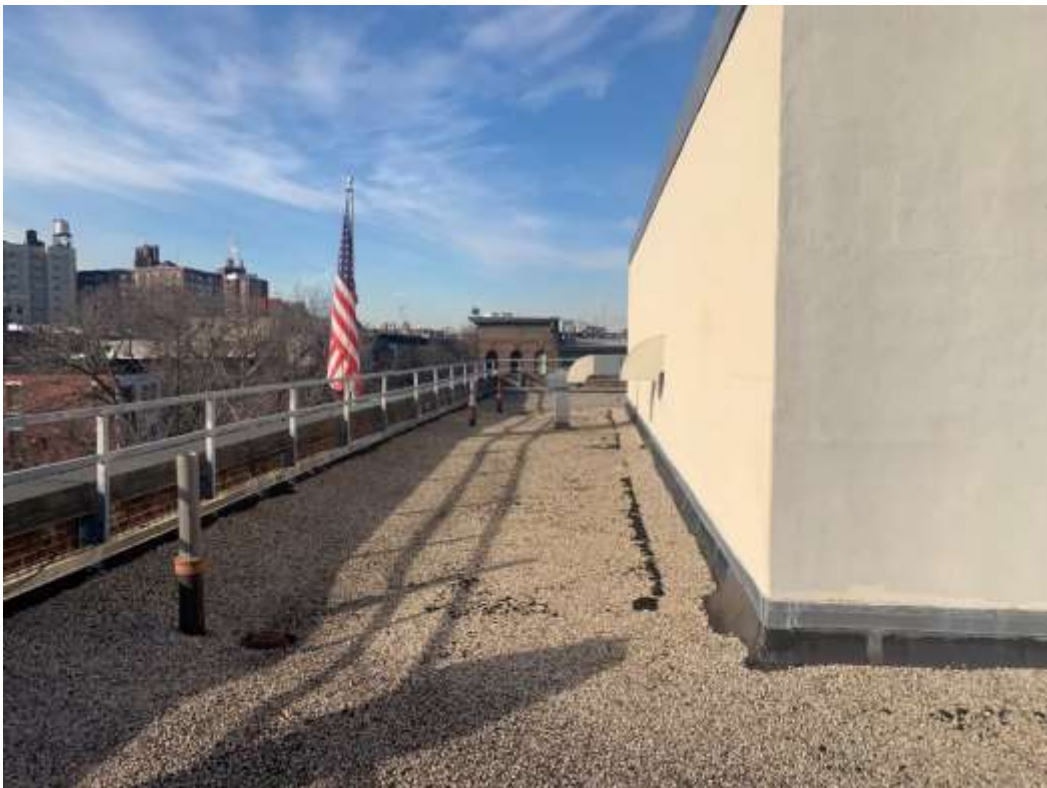
Photo R10 – View of Roof and Southwest Bulkhead, facing West.
