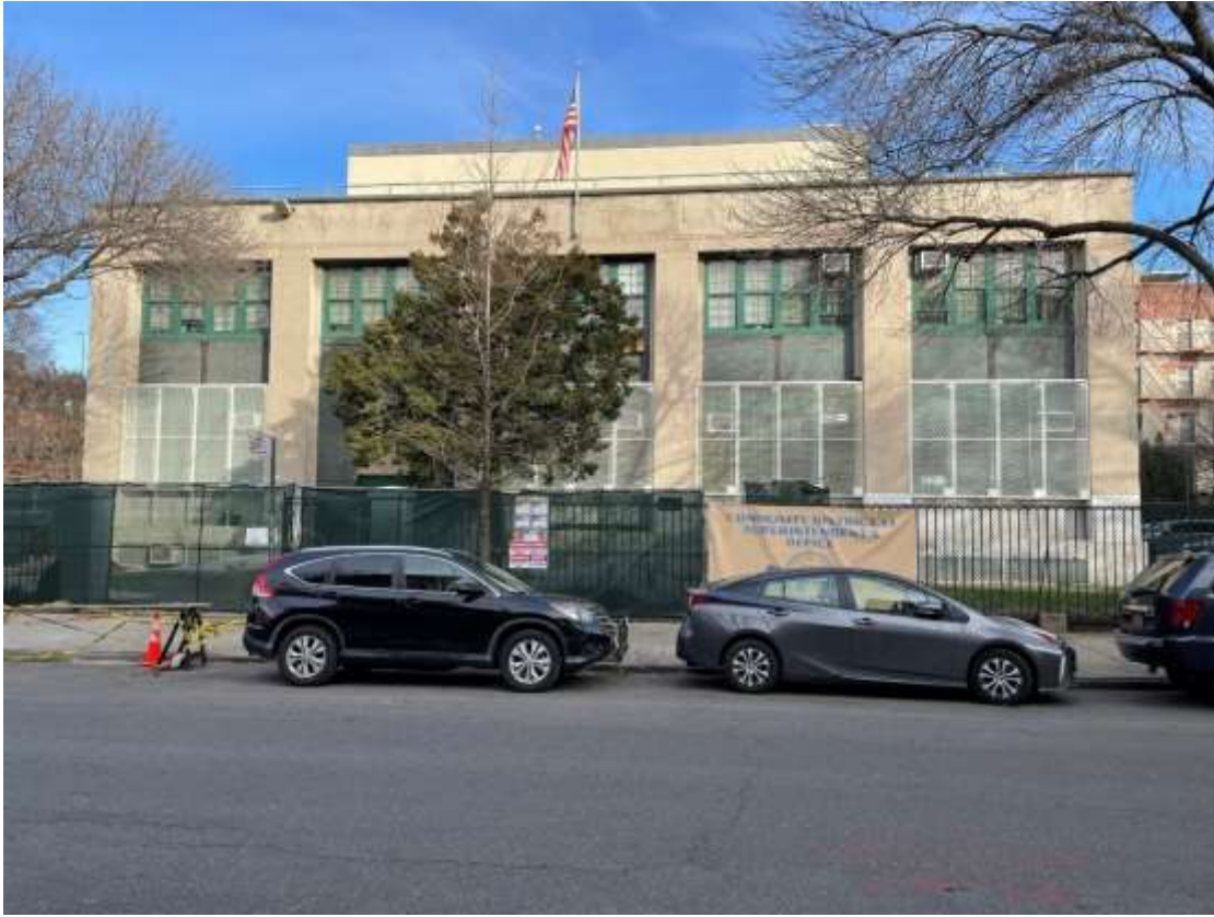
Photo M01 – View along Park Place – South Façade.
