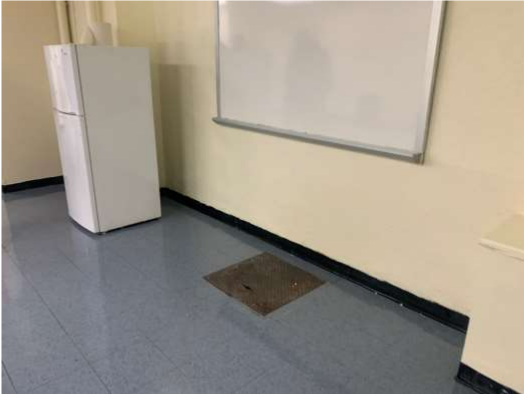
Photo A23 – Floor hatch at Room B3A.
