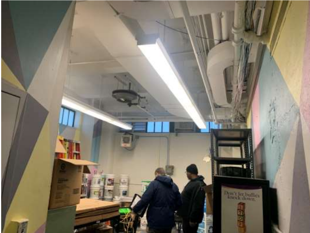
Photo A03 – View at storage room B2A.
