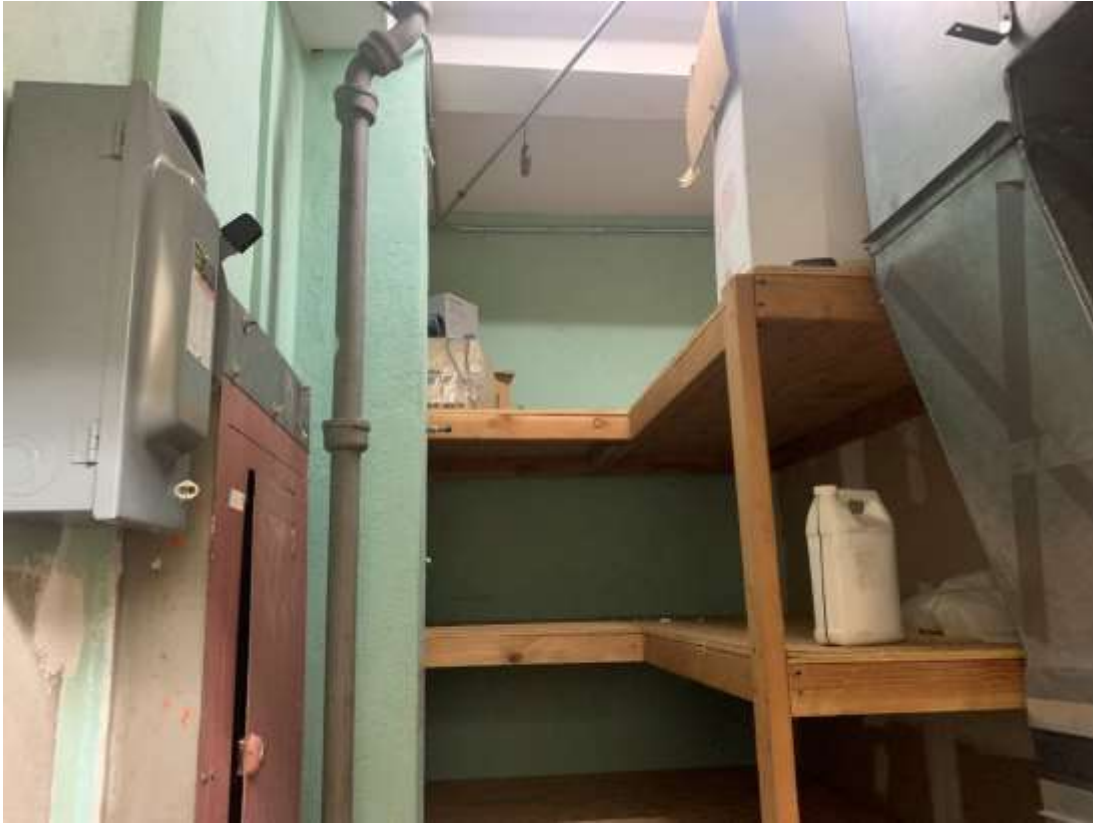
Photo A34 – View of Storage Room at Bulkhead.
