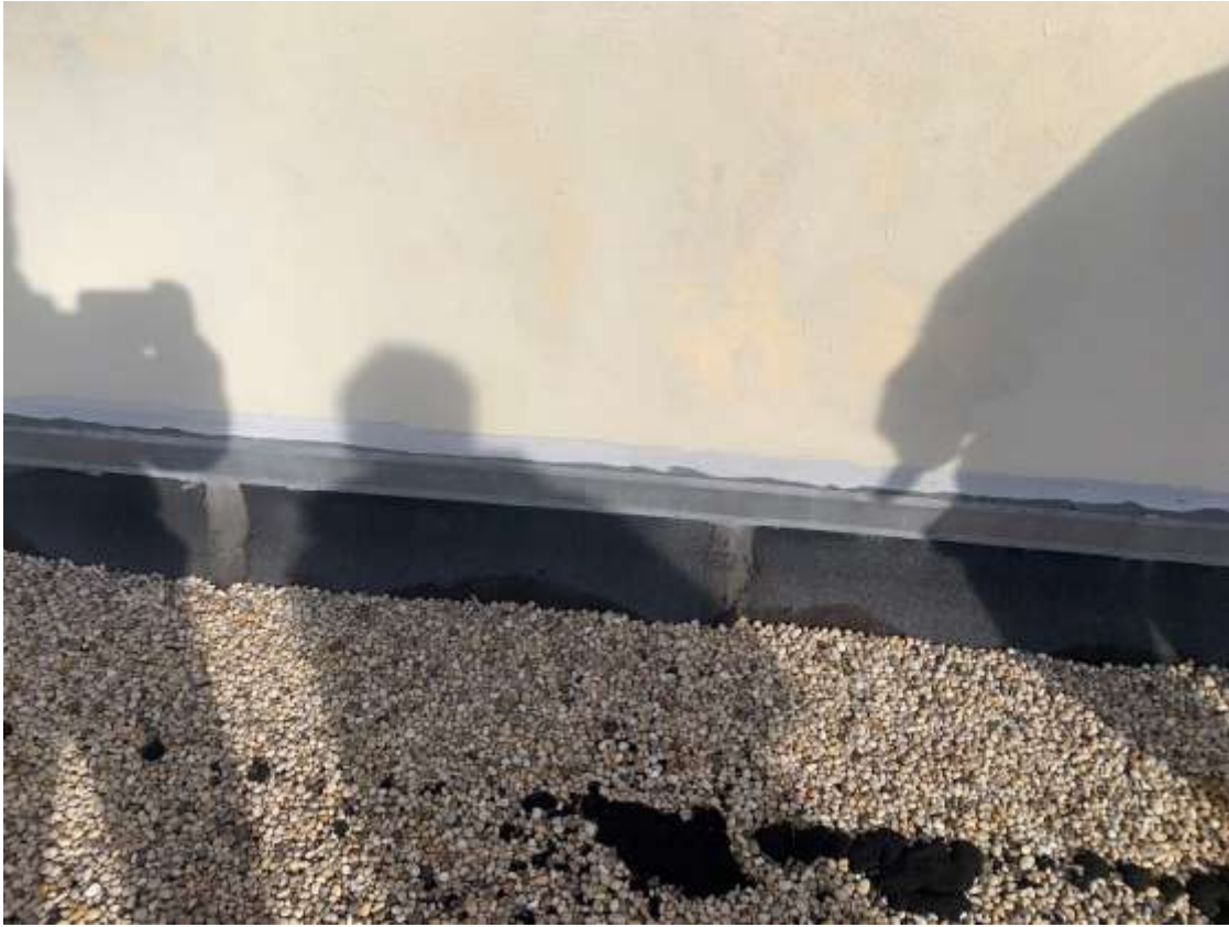
Photo R05 – Roof flashing is in good condition.
