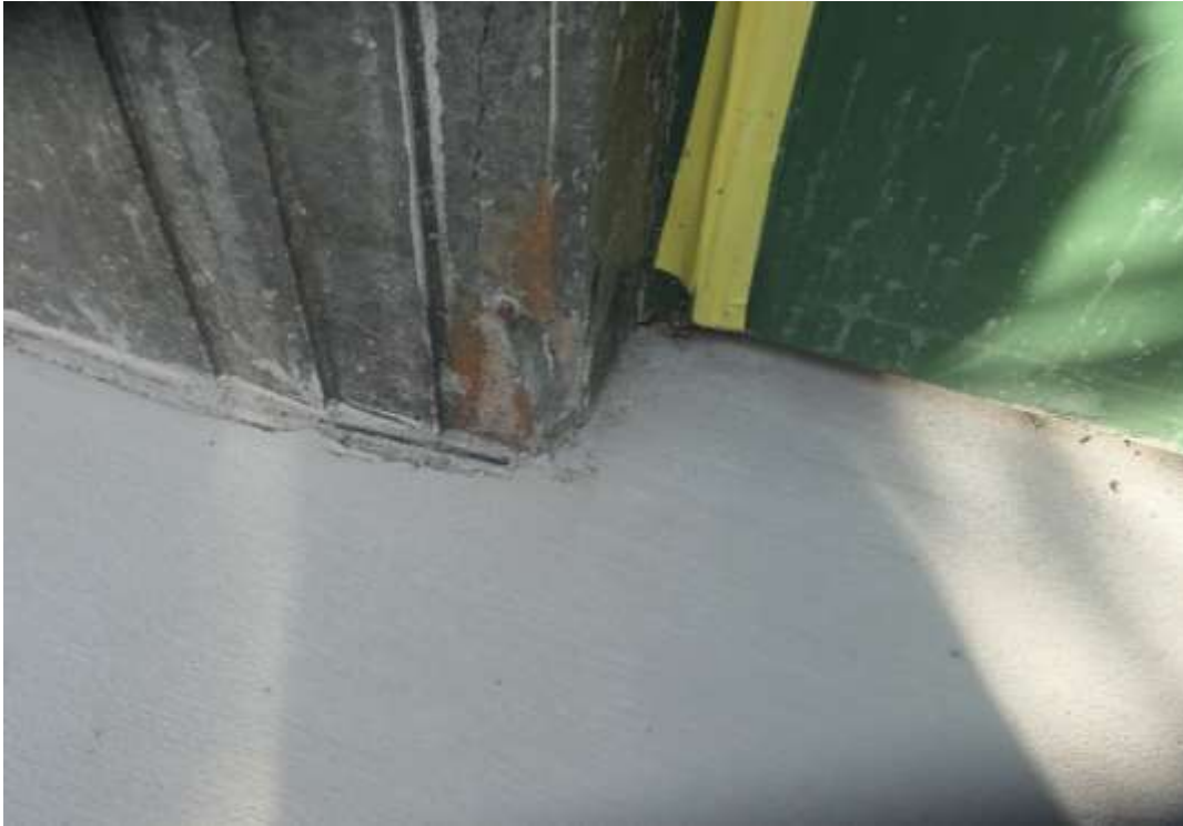
Photo M13 – Close detail to the missing stone and crack in granite.
