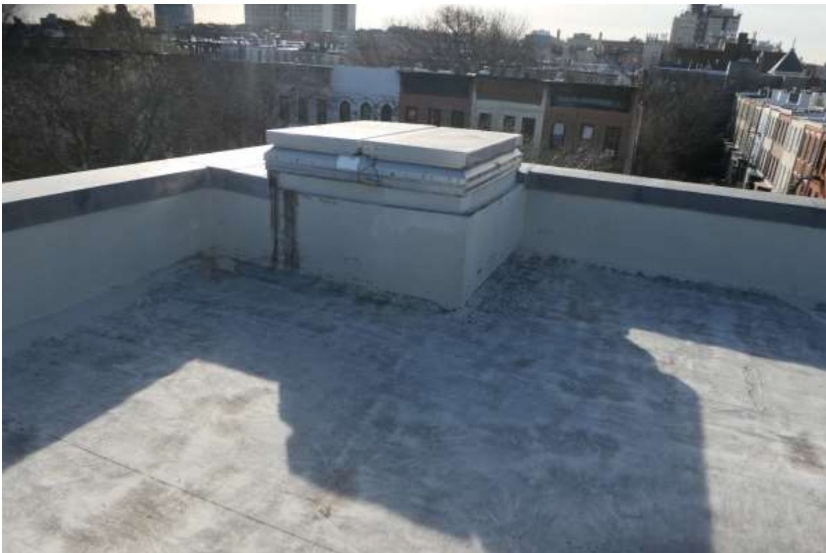
Photo R18 – Roof hatch at Bulkhead roof is in good condition.
