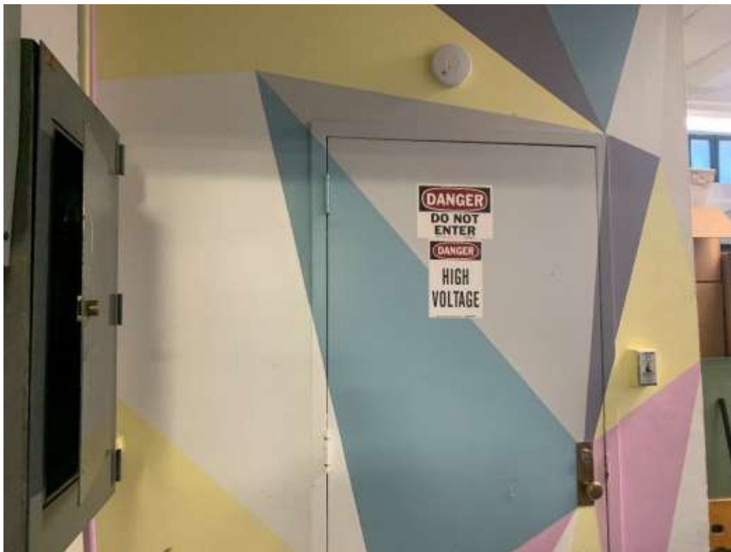
Photo A04 – View of electrical closet's door at Room B2A.
