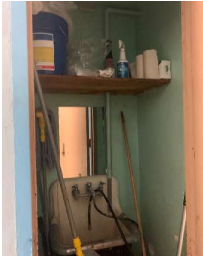
Photo A11 – Closet next to restroom at Basement Level B5.
