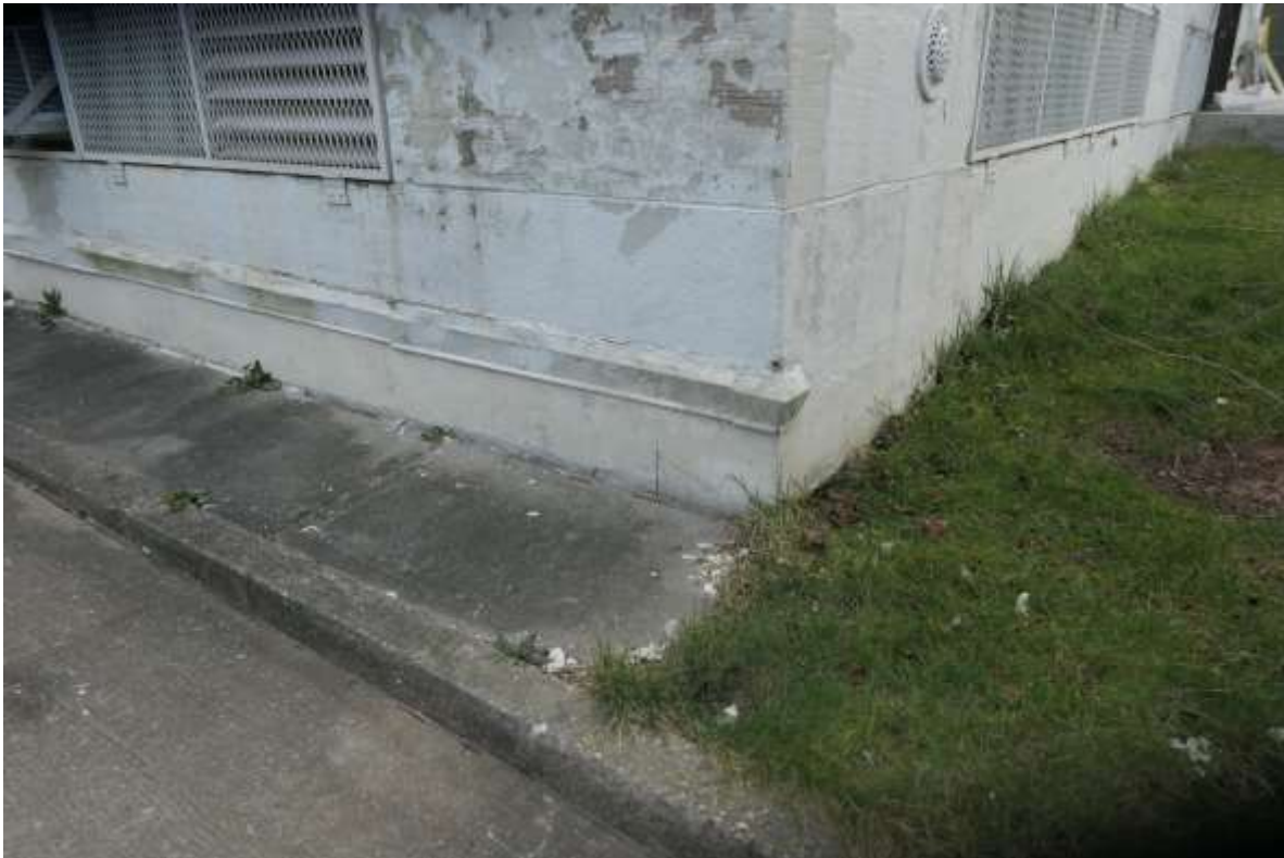
Photo S12 – Sidewalk next to parking driveway is in fair condition.
