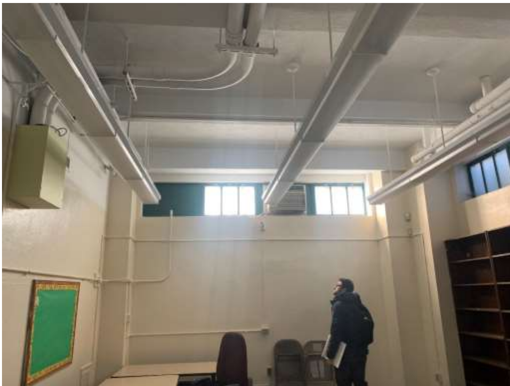
Photo A14 – View of Library B1 view along South Façade.
