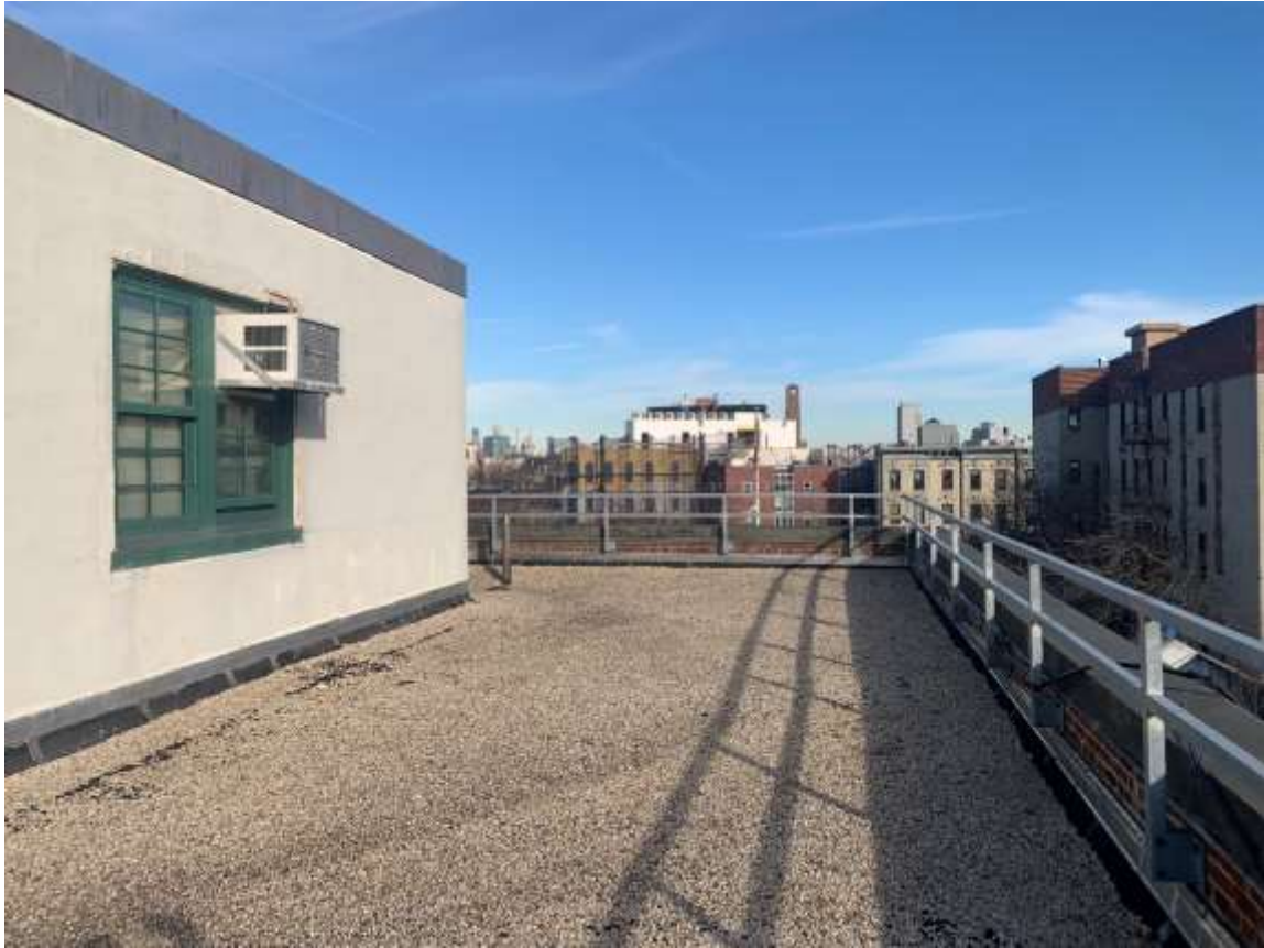
Photo R11 – View of Roof and East Bulkhead façade, facing North.
