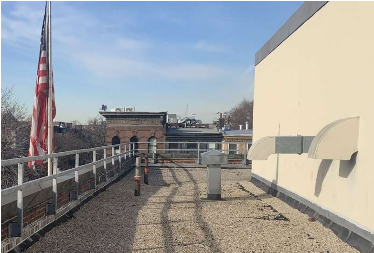
Photo R08 – View of Roof and South Bulkhead façade, facing West.
