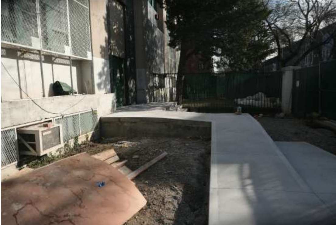
Photo S01 – Existing ramp at main entrance.
