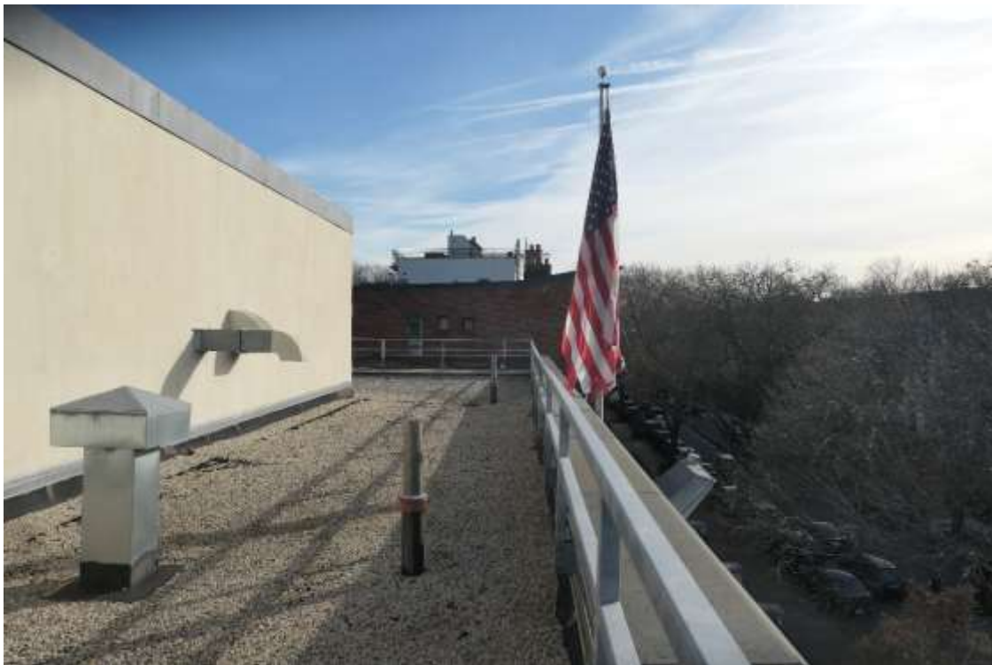
Photo R04 – View of Roof and South Bulkhead façade, facing East.
