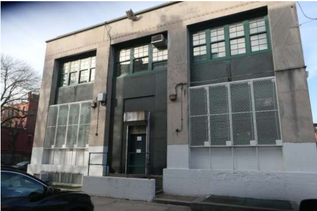
Photo M02 – View from parking lot – East Façade.
