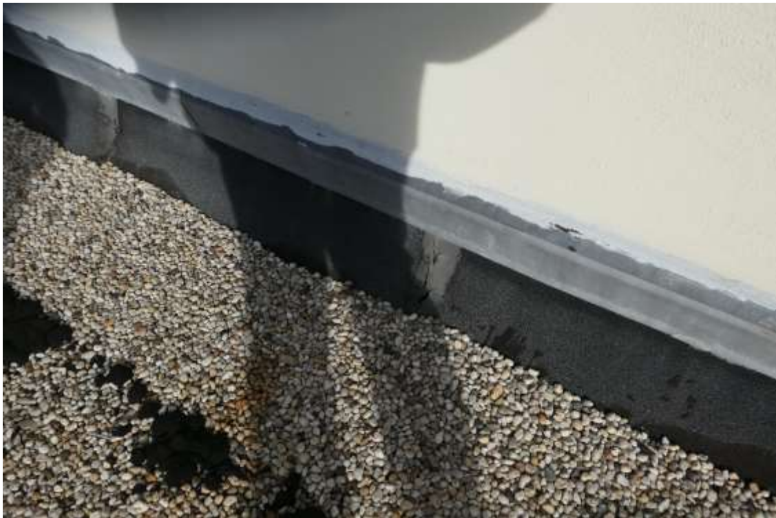
Photo R06 – Roof flashing is in good condition.
