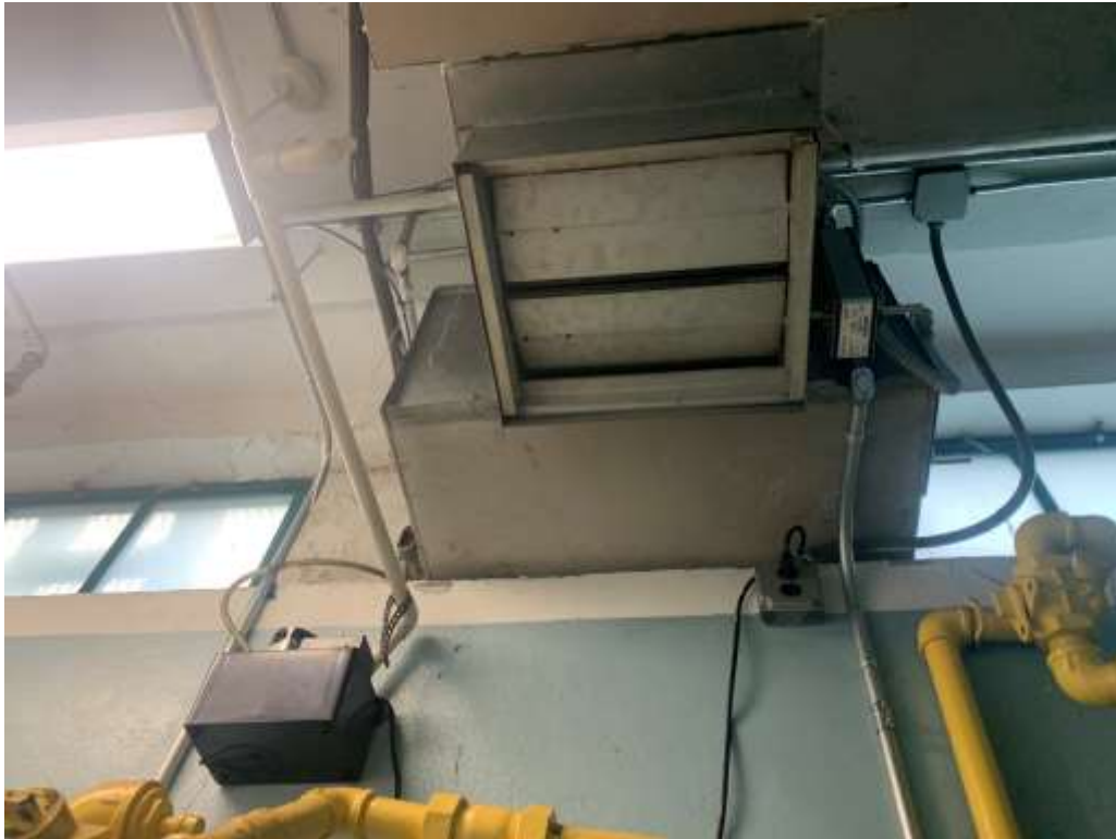
Photo A27 – View of Storage Room B3C.
