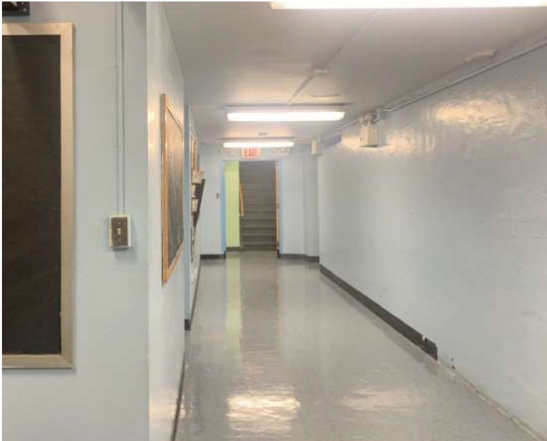
Photo A18 – View of hall towards Stair #3
