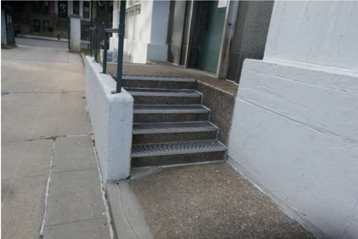
Photo S07 – Stairs are in good condition.
