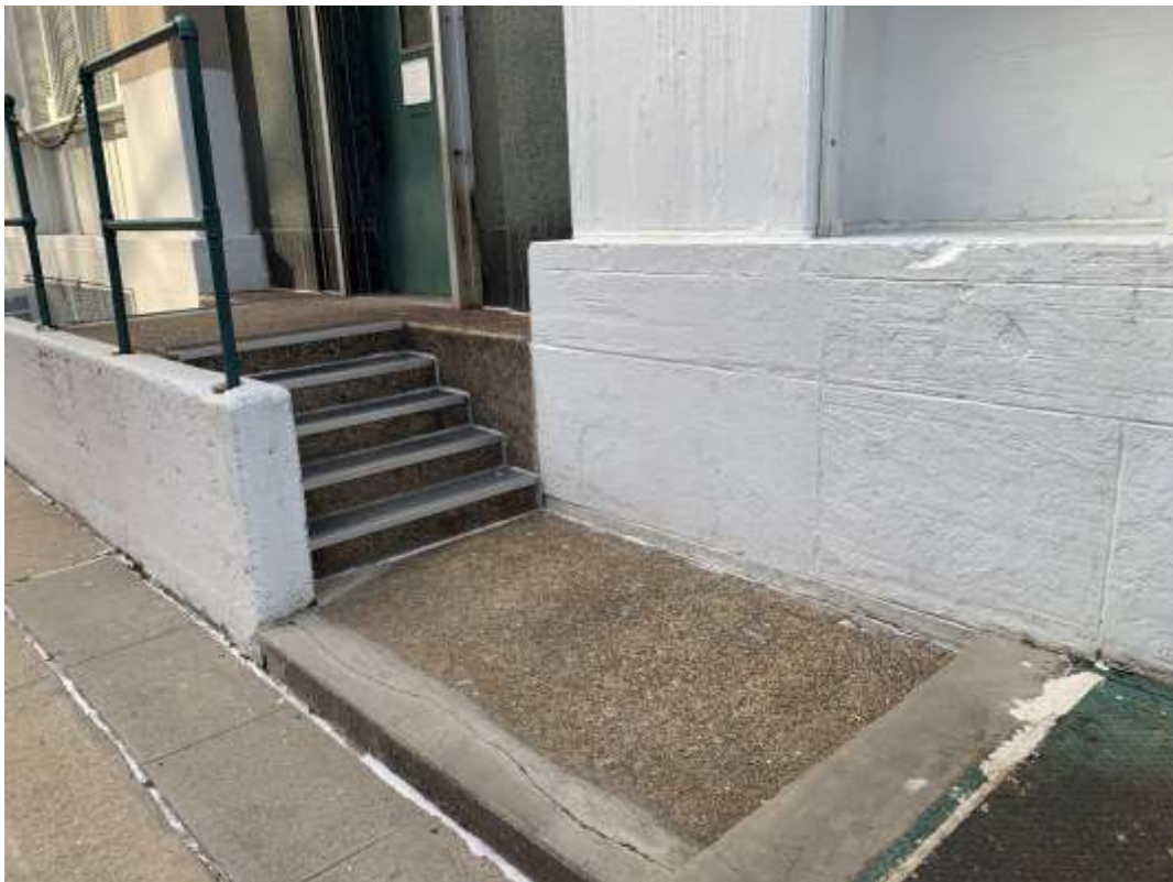
Photo S06 – Stairs to Entry #2 at East Façade.
