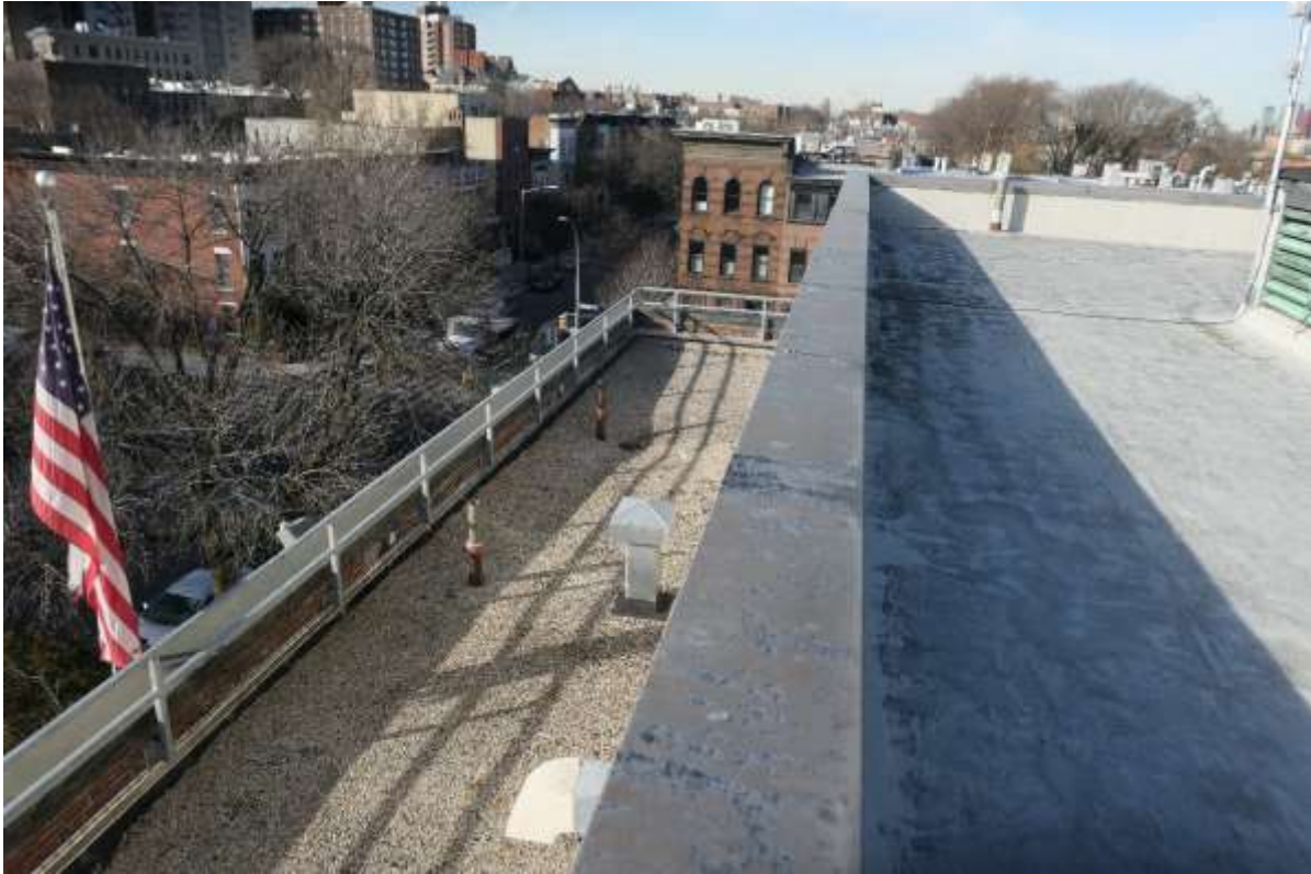
Photo R17 – View of Roof and Bulkhead roof facing North.
