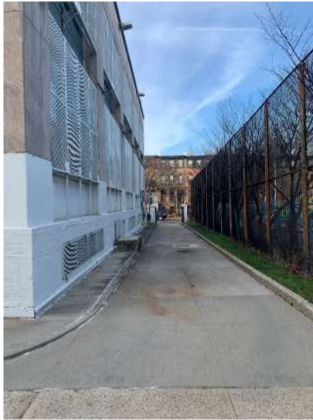
Photo M29 – View along back entrance – North Façade.
