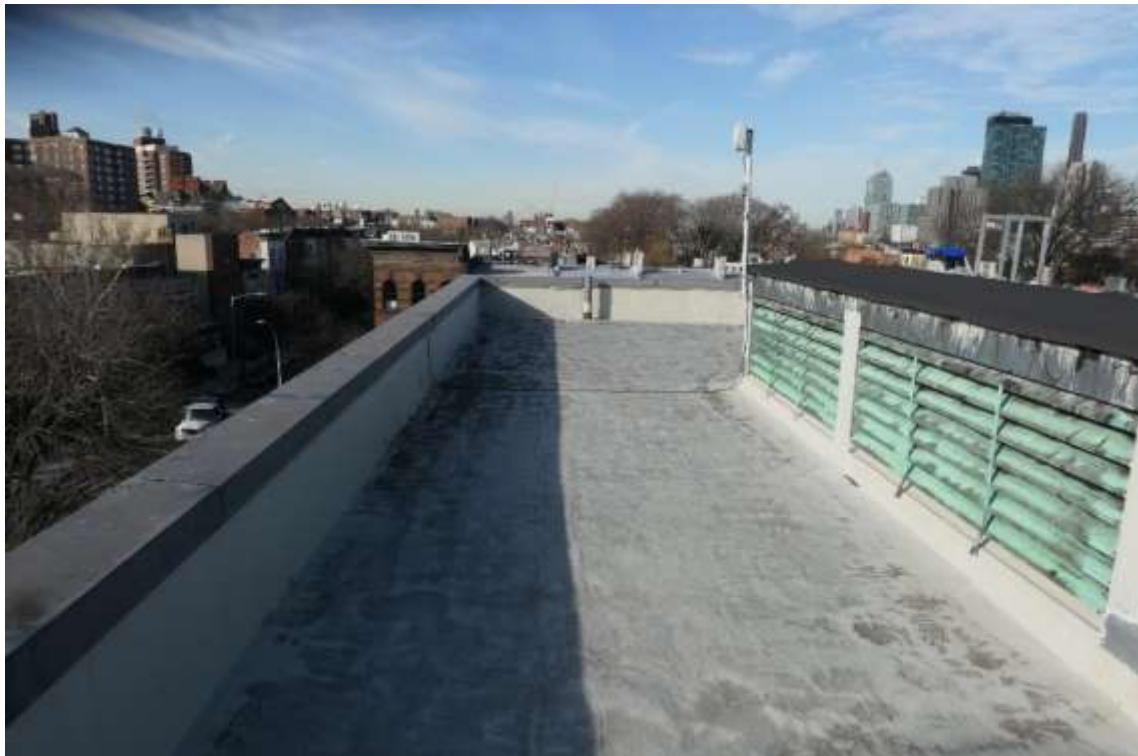
Photo R16 – View of bulkhead roof facing West.
