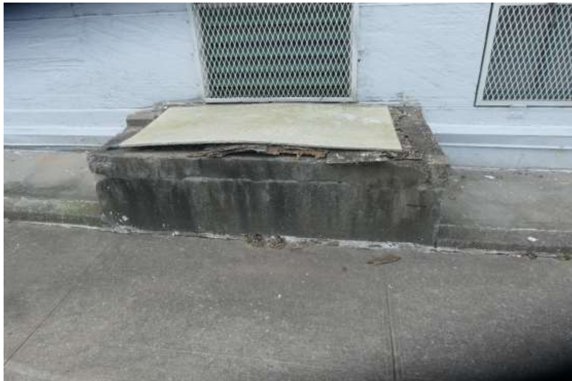
Photo S10 – Areaway is in fair condition.
