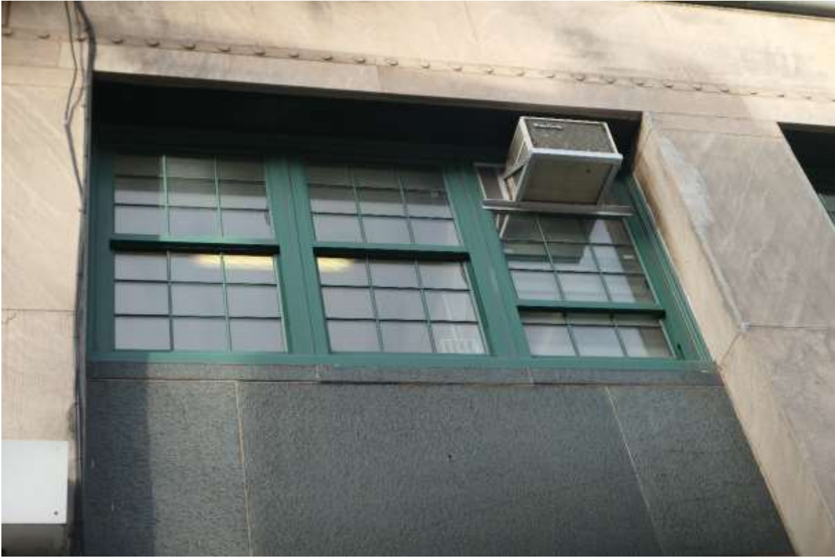
Photo M27 – Double hung windows and ACs are in good condition.
