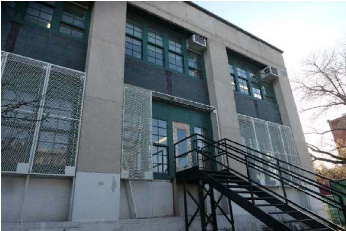
Photo M44 – Temporary access at West Façade.
