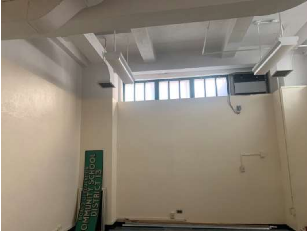
Photo A32 – View of Room B3B.
