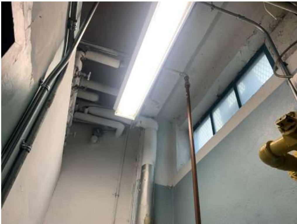
Photo A29 – View of Storage Room B3C.
