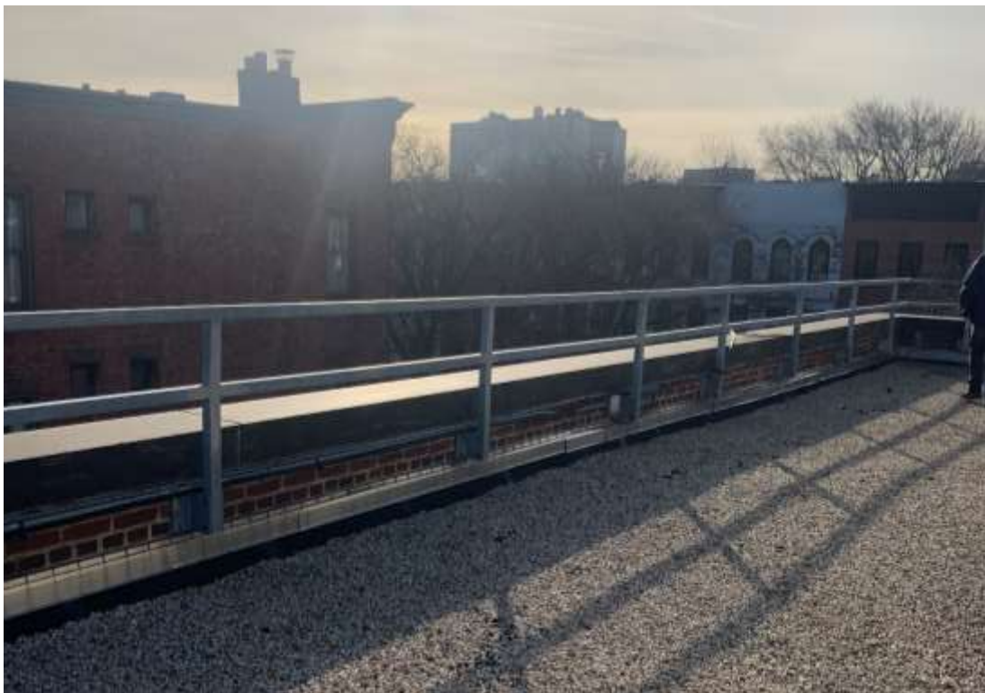
Photo P06 – Roof Barrier is in good condition.
