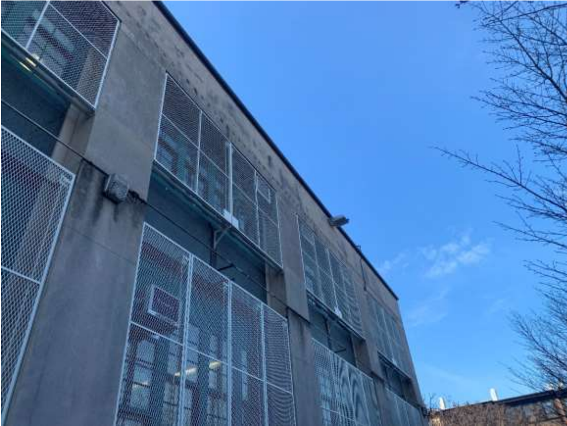
Photo M33 – Window guards are in good condition – North Façade.
