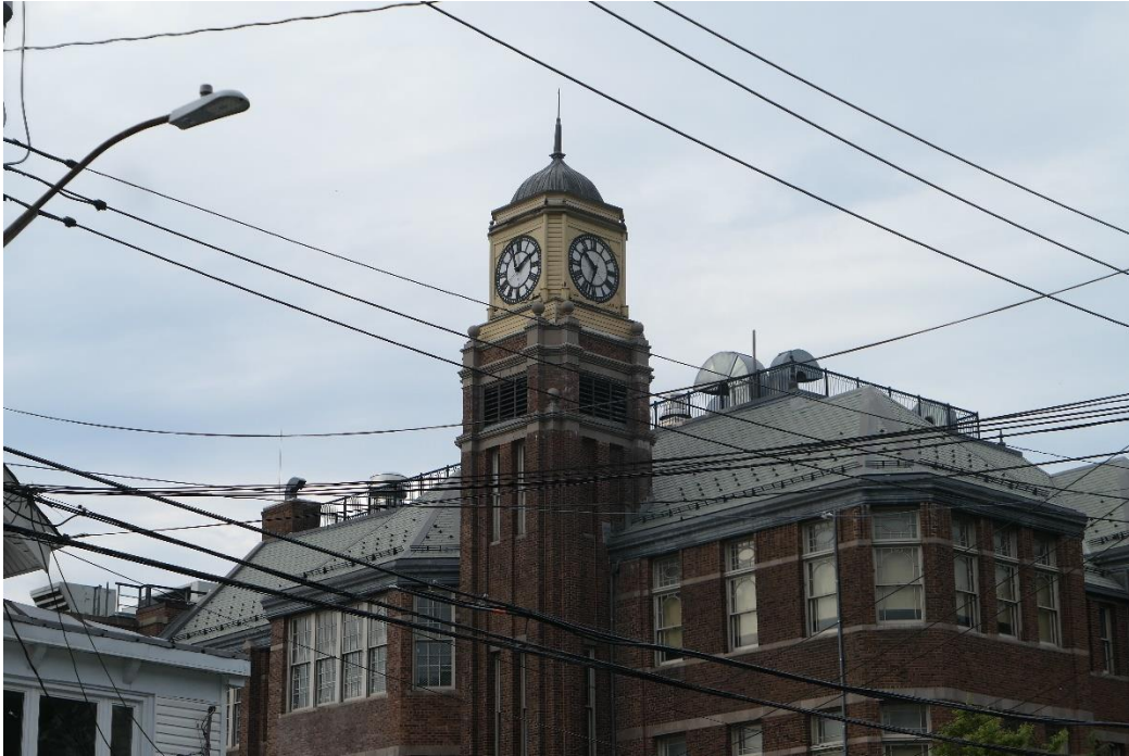
Photo 11 – Clock Tower view from St. Paul’s Ave.
