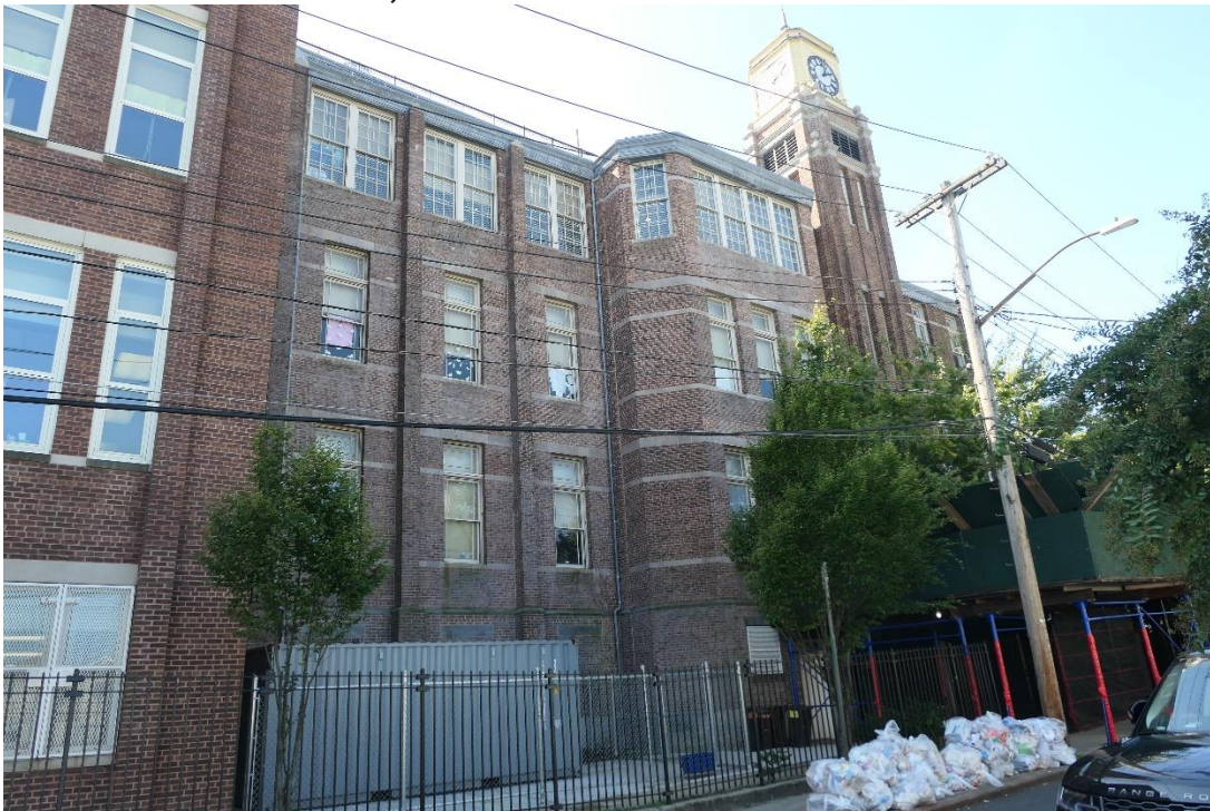
Photo 2 – North elevation, original building at Grant St.
