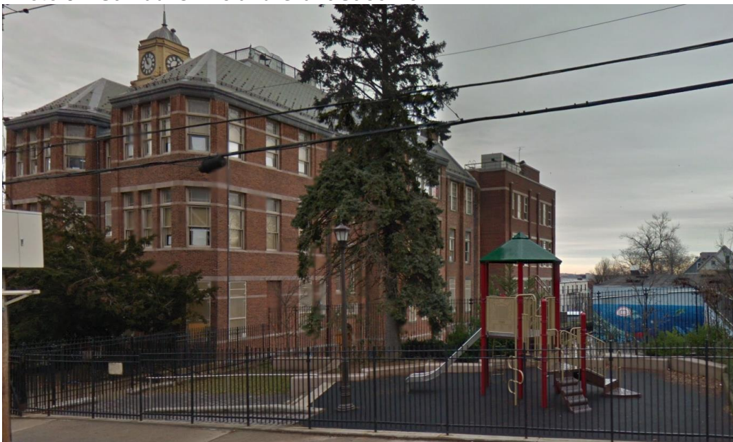
Photo 6 – South elevation and playground at St. Paul's Ave.
