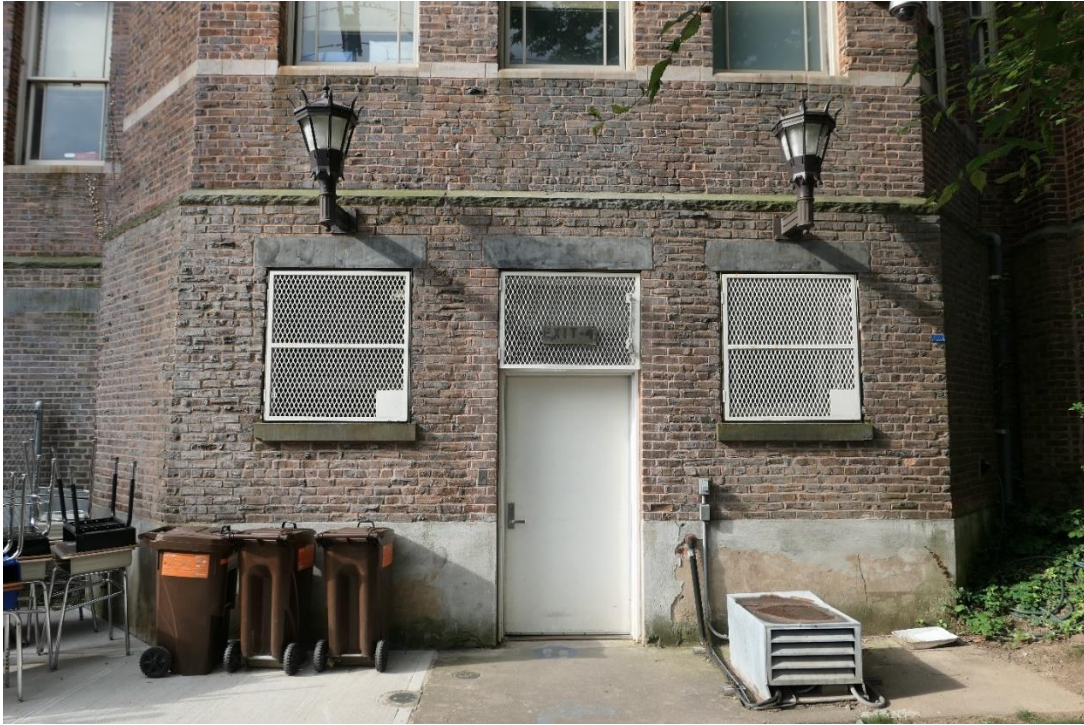
Photo 9 – Lateral service door at Grant St.
