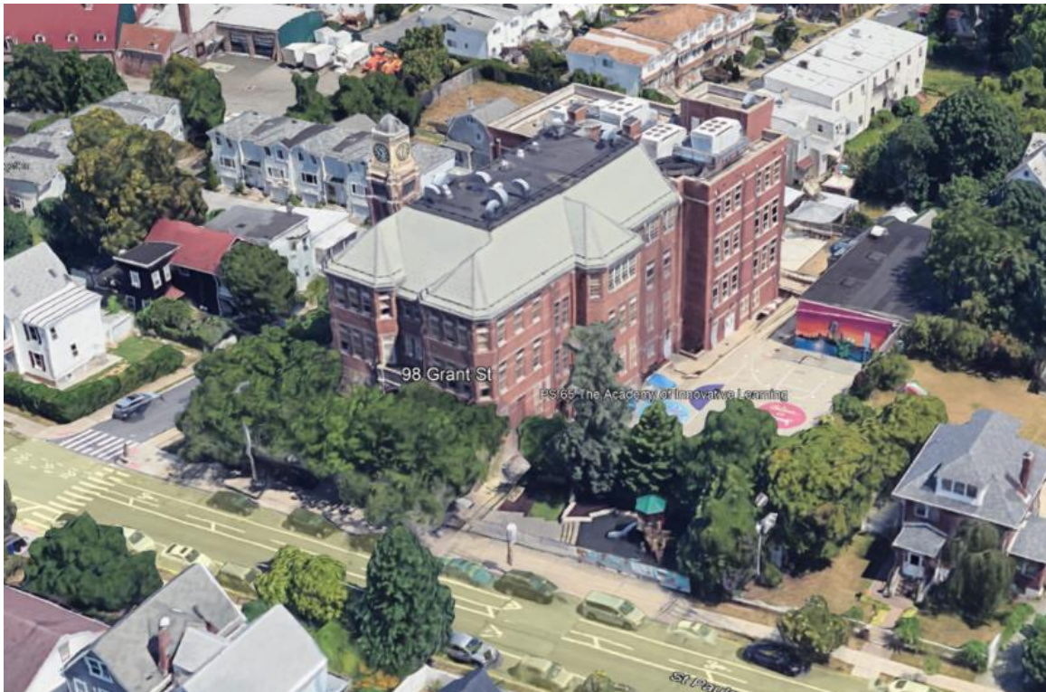
Aerial View – Southwest
