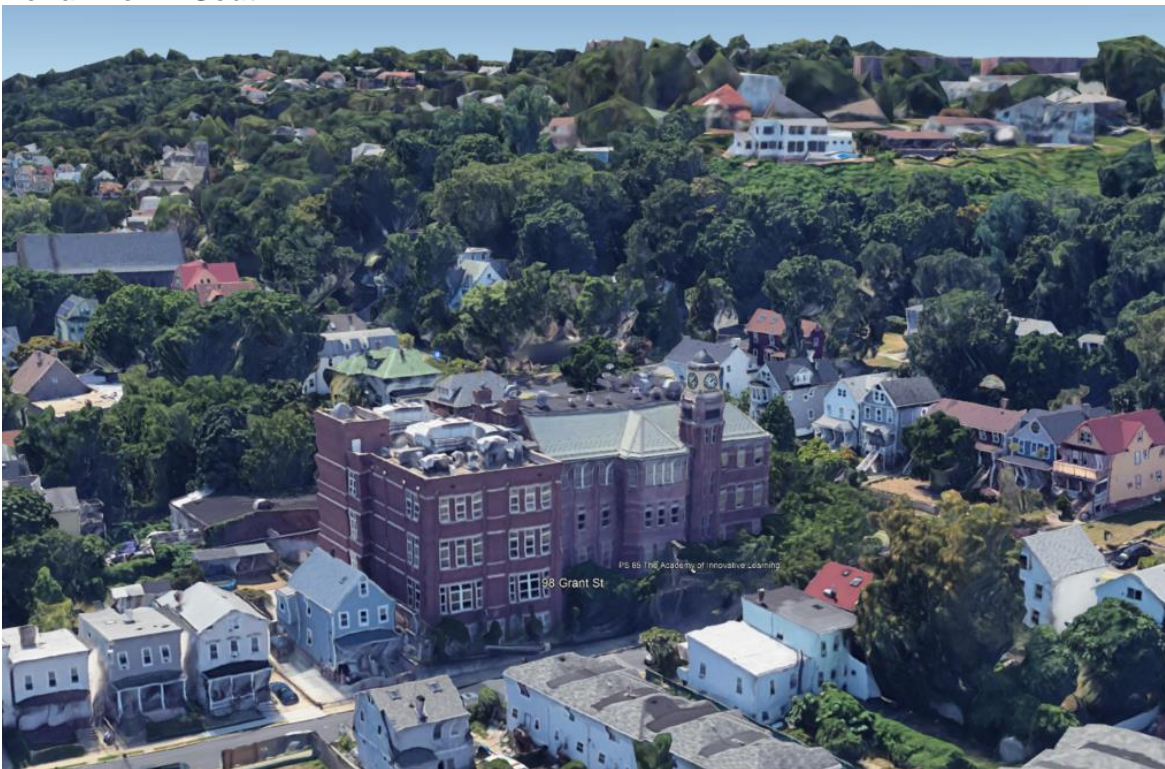
Aerial View – North
