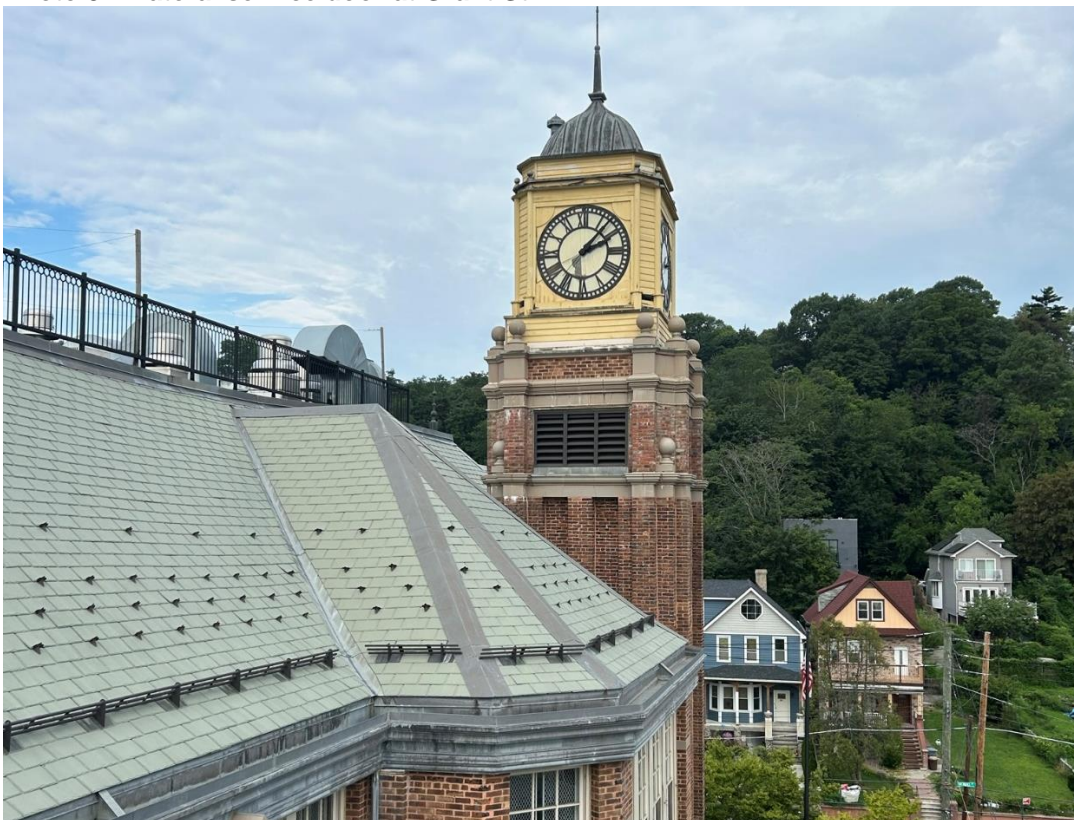
Photo 12 – Clock Tower and Roof view from Grant St.
