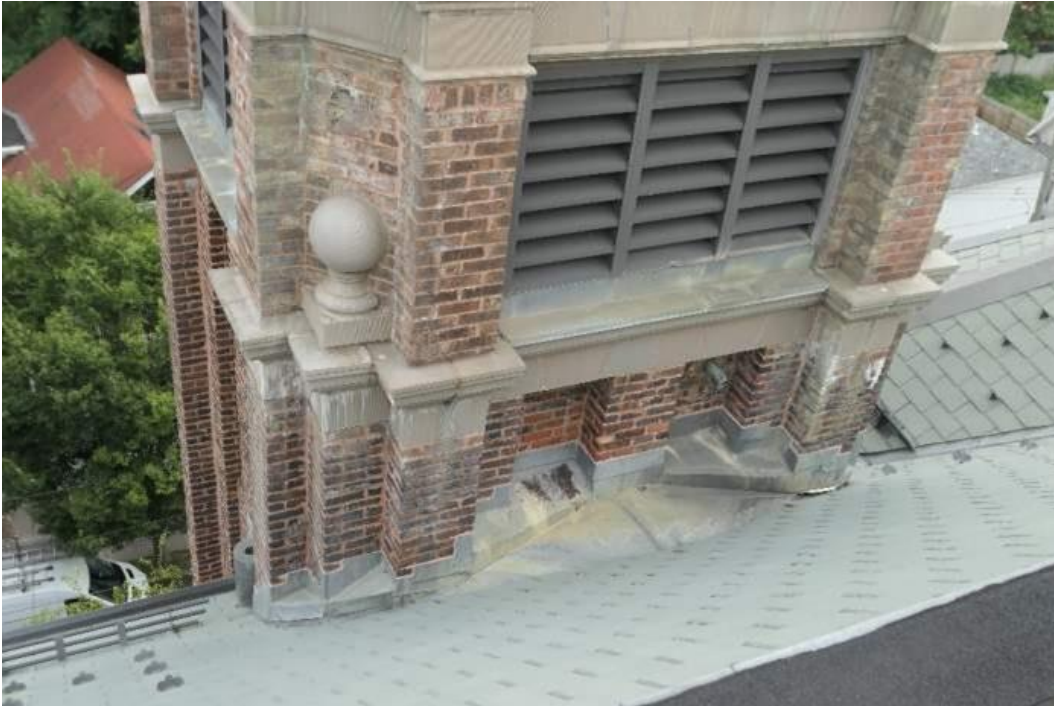
Photo 5 – Masonry, flashing and roofing below cupola in good condition.
