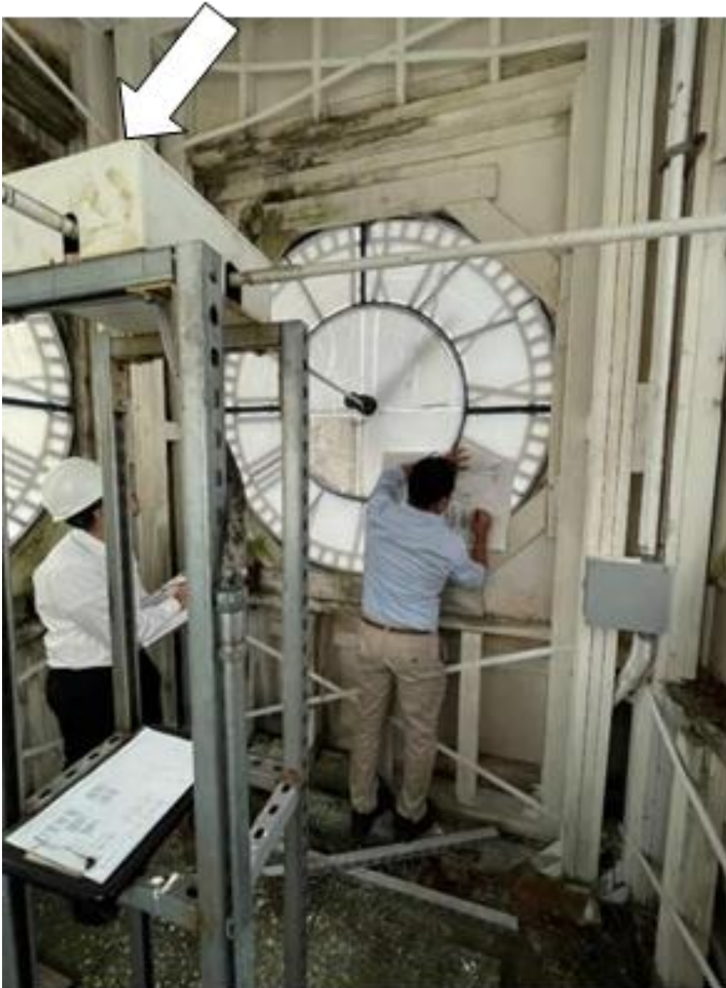
Photo 12 – Central clock mechanism controls hands on all four faces. Clocks are not working.
