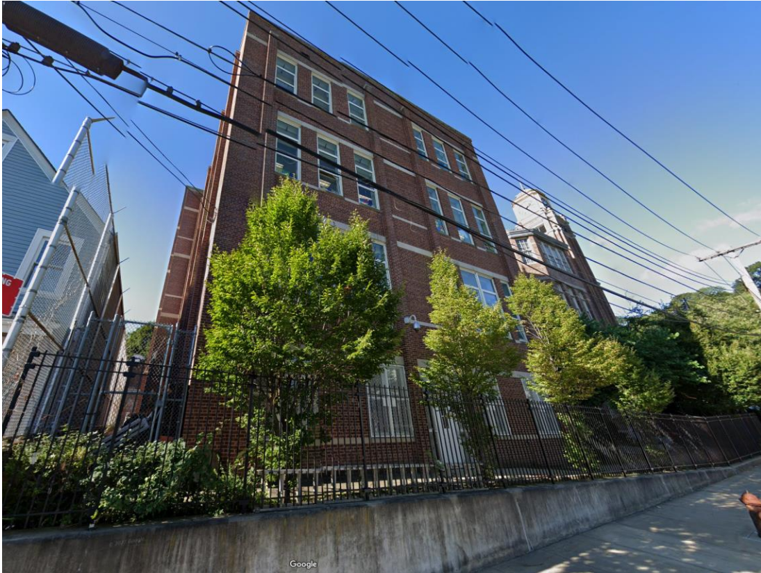
Photo 3 – North elevation, addition at Grant St.
