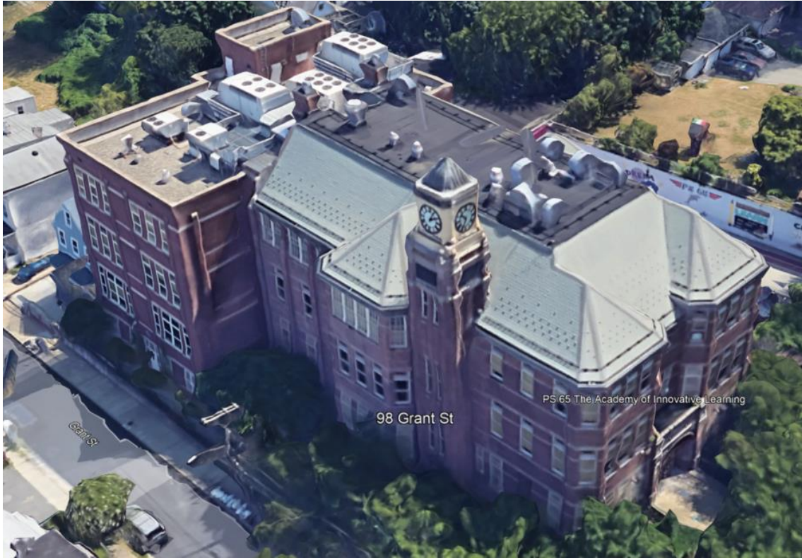
Aerial View – Clock Tower
