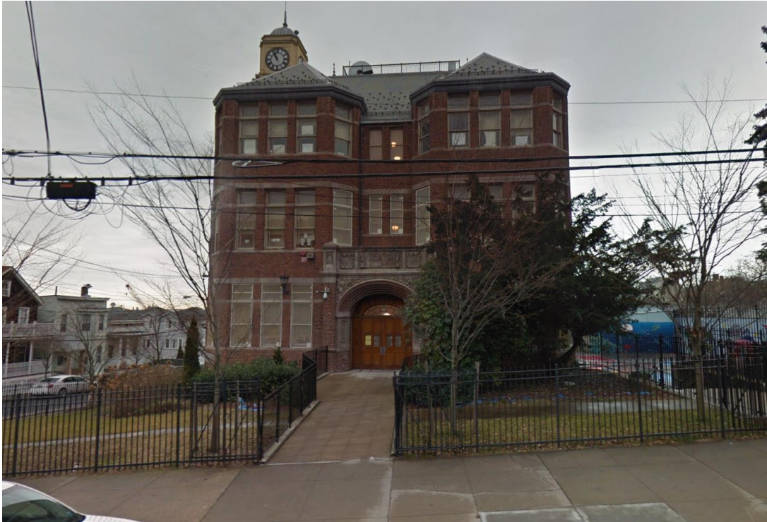
Photo 1 – West elevation, main access at St. Paul's Ave.
